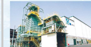
Mizue Recycling Plant
